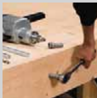
WB system for reinforcements in glulam timber construction
