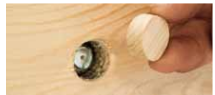
7. Cover hole with end-grained wooden plug.
