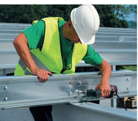
Both the connection of longitudinal joints and the attachment of purlins is performed in a single operation. The TDBL thread forming fastener is inserted in the punched hole and installed fatigue-free using a battery-powered impact screw gun: **simple**, **fast** and **secure**.
